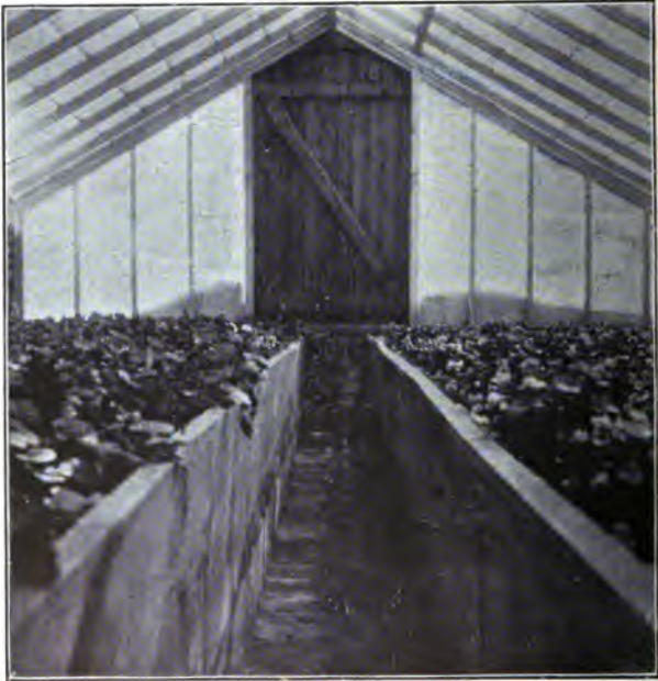
16.—Interior of twelve foot house, showing method of constructing south end and door.
